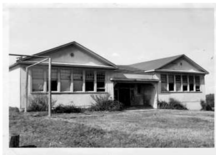
East side facade of Port Orford High School
