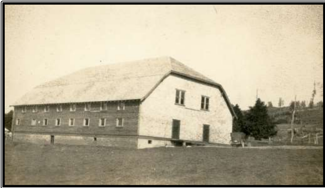
ORIGINALLY, THE GYM DID NOT HAVE A SOUTH SIDE PORCH.
