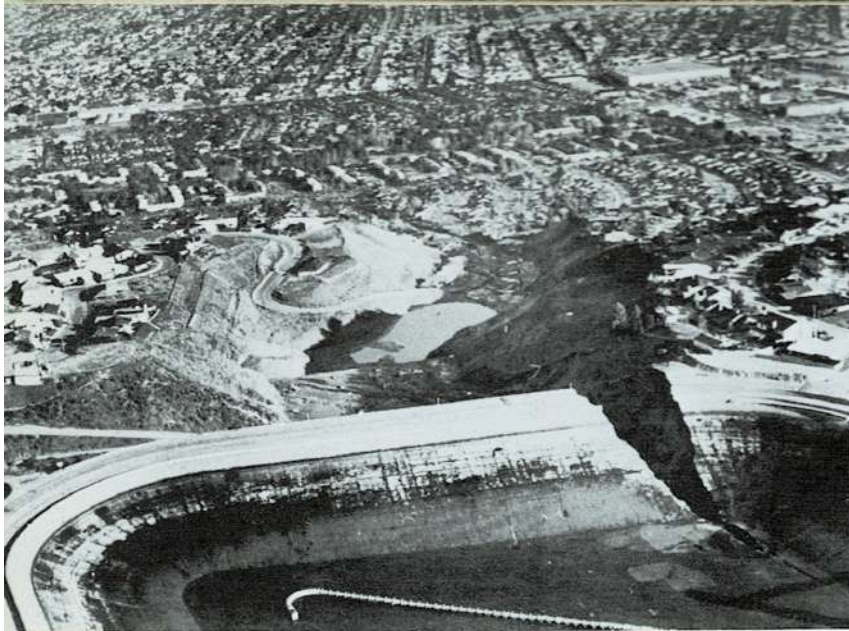
In Los Angeles, Baldwin Hill Reservoir cracked, then broke releasing a torrent which wrecked hundreds of evacuated homes, but produced few casualties.
